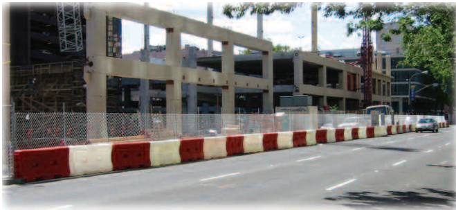
The TrafFix Water-Wall used as a Longitudinal Barricade along a job site.
